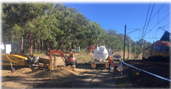
Sydney Trains electrical and communications upgrade
