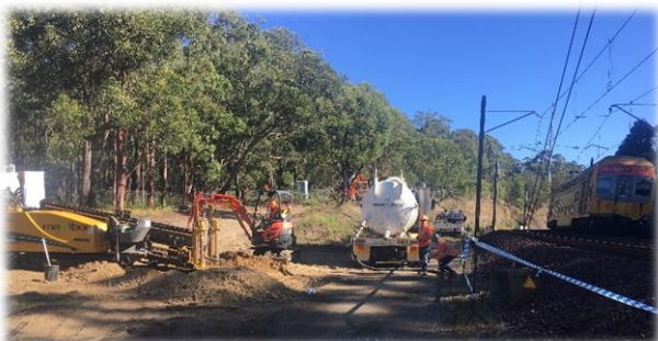
Sydney Trains electrical and communications upgrade
