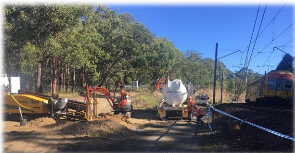
Sydney Trains electrical and communications upgrade
