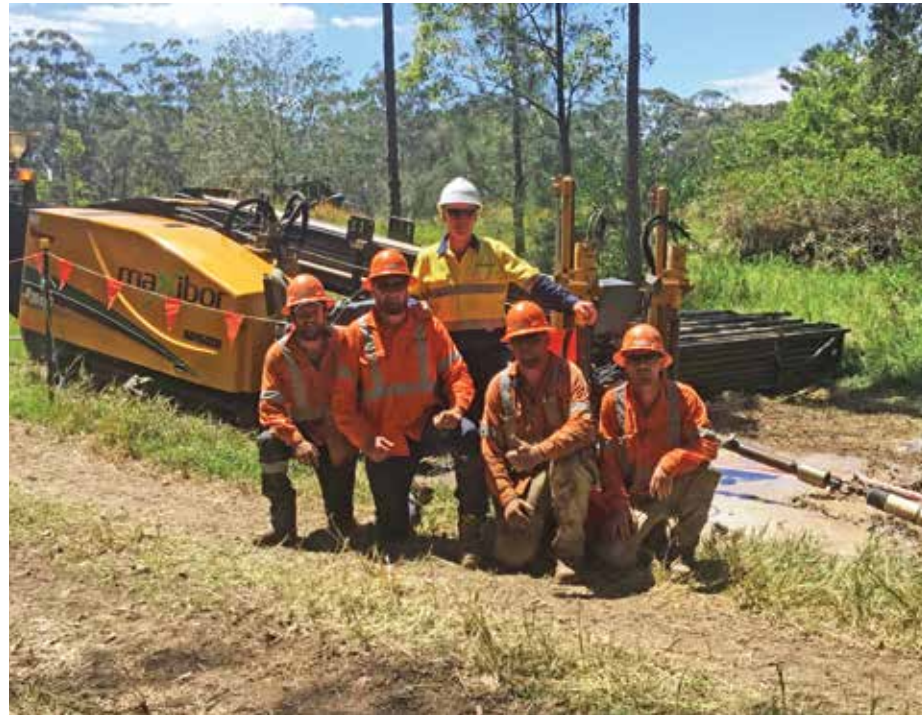
The Maxibor team at the Gumma Road project site.
